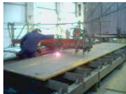
Cutting the frames 13/9/04
