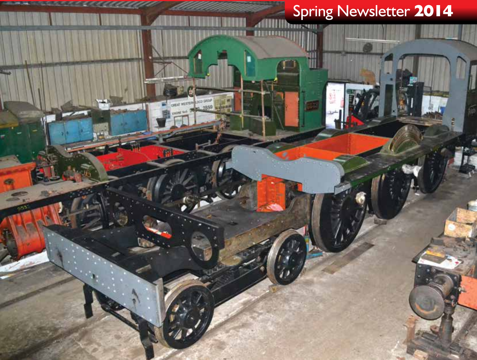
The newly refurbished bogie from No. 5952 Cogan Hall is situ under the frames of No. 6880 Betton Grange , but cannot be fitted permanently until the new cylinders are made and in position. CHRIS MOORE
